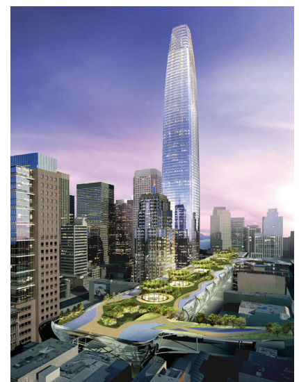
The center’s first phase will include a five-story bus terminal stretching across four blocks and a rooftop park comparable to New York’s High Line.
